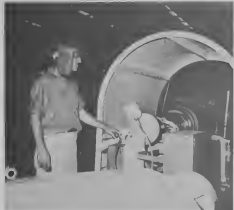
MACHINIST USES face shield for maximum eye protection for work on specific machines. MACHINIST TA usa capa pa cara pa mayor proteccion di wowo ora ta traha cu cierto mashin.
